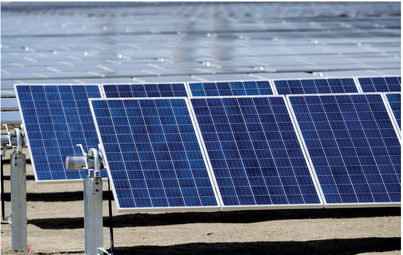
Solar panels covering 900 acres are seen at the Comanche Solar facility in Pueblo, Colorado April 6, 2016. REUTERS/Rick Wilking
